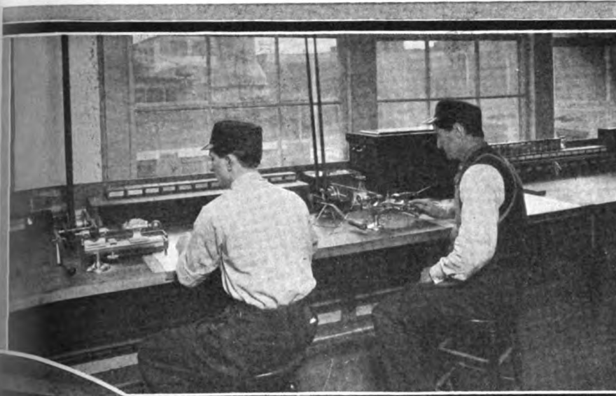
Corner of the Watch Lathe Department Where Needle Valves, Nozzles and Other Small Parts are Made to Great Accuracy
